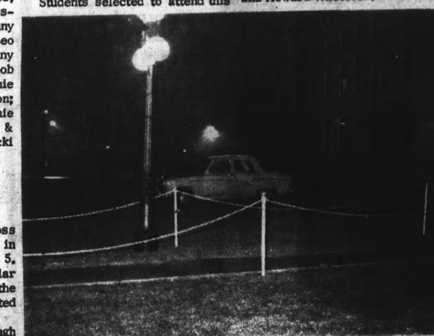
Construction Started On New Parking Lot
