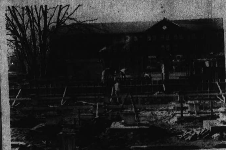
1959 - Construction of Morrison Hall
