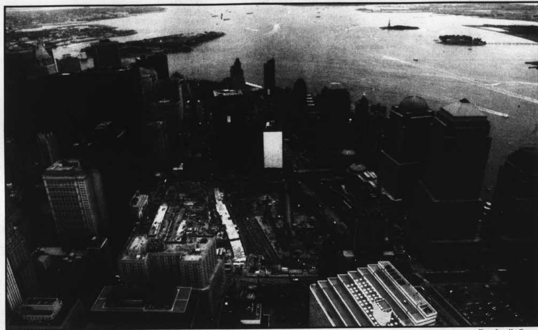
The site where the World Trade Center once stood has moved into the construction phase.
