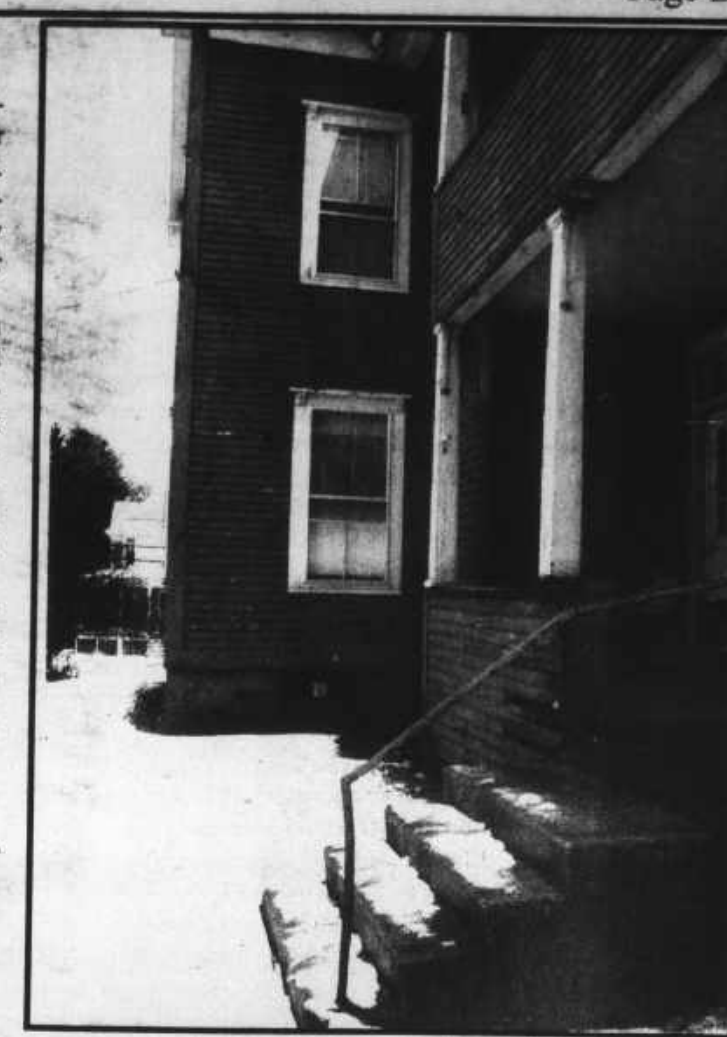
Some of the apartment buildings in Keene are in pretty bad shape, like this one on Roxbury Street.
