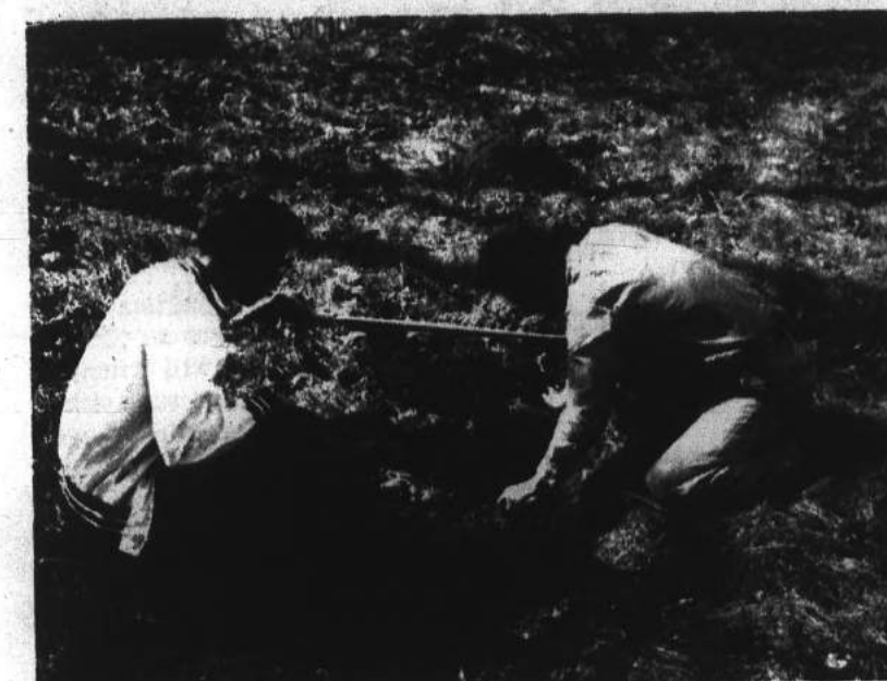
Digging on Connecticut River
