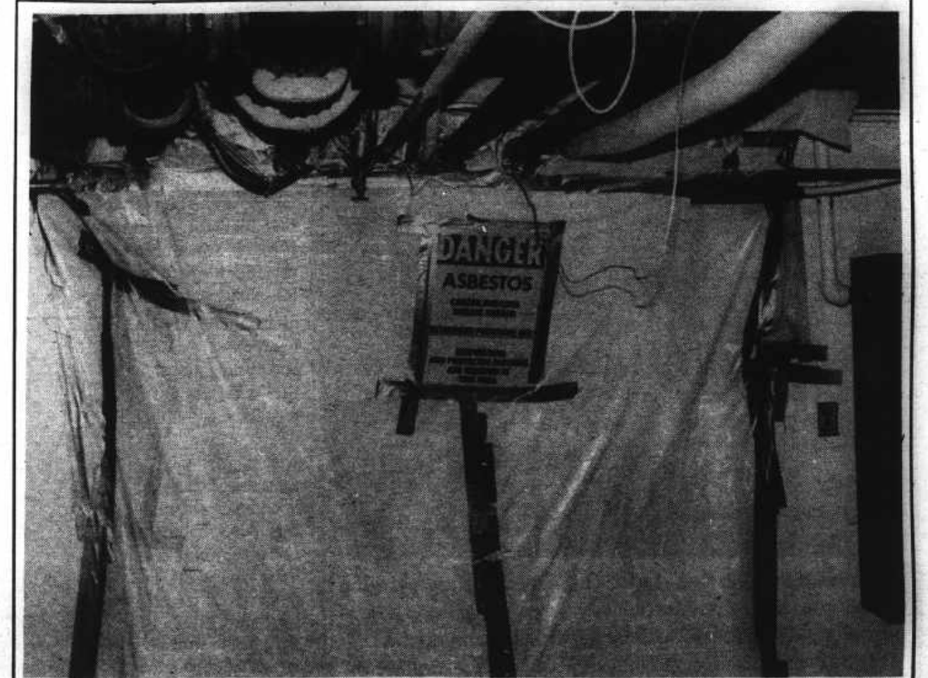
Workers sealed off this section of the Elliot Hall basement during the removal of asbestos this summer.
