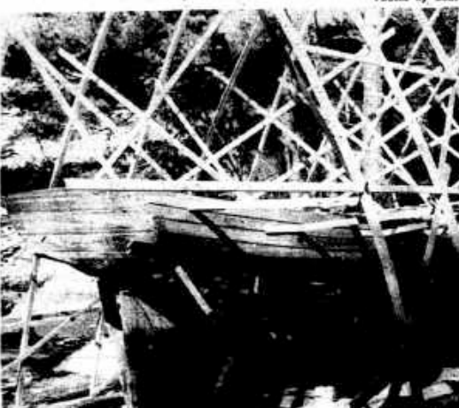
Above are two visual perspectives of the 'Epic', LIVE's schooner which will be completed by students of the program within three years. The boarding surrounding the boat frame is the beginning of a dome which will protect the boat from damage during storm weather.
