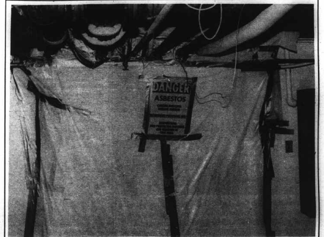
Workers sealed off this section of the Elliot Hall basement during the removal of asbestos this summer. Equinox/Scott McPherson
