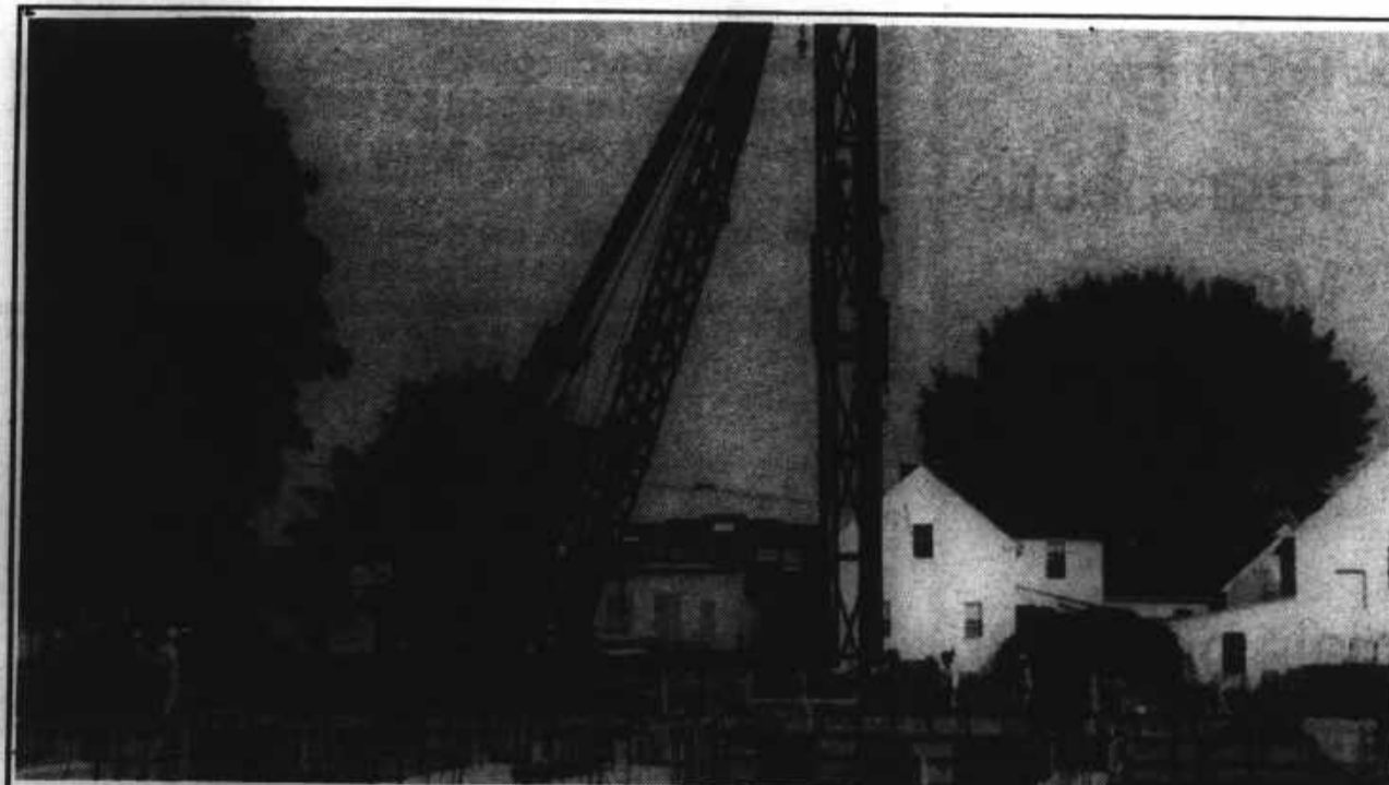
September of 1988 saw the ground breaking for the new residence hall. Here, piles are driven into the ground to help secure the foundation.
