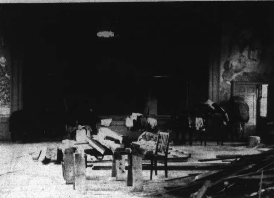
THEATER IN THE RAW — Work shown above is the first stage of the renovation of Parker Hall into an adequate college theater. The redmen will soon be vanishing.
