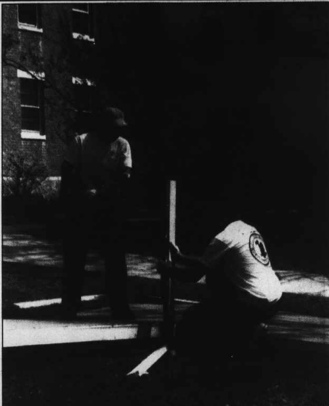
Bob Dumond and Steve Schnyer work on building the graduation platform.
