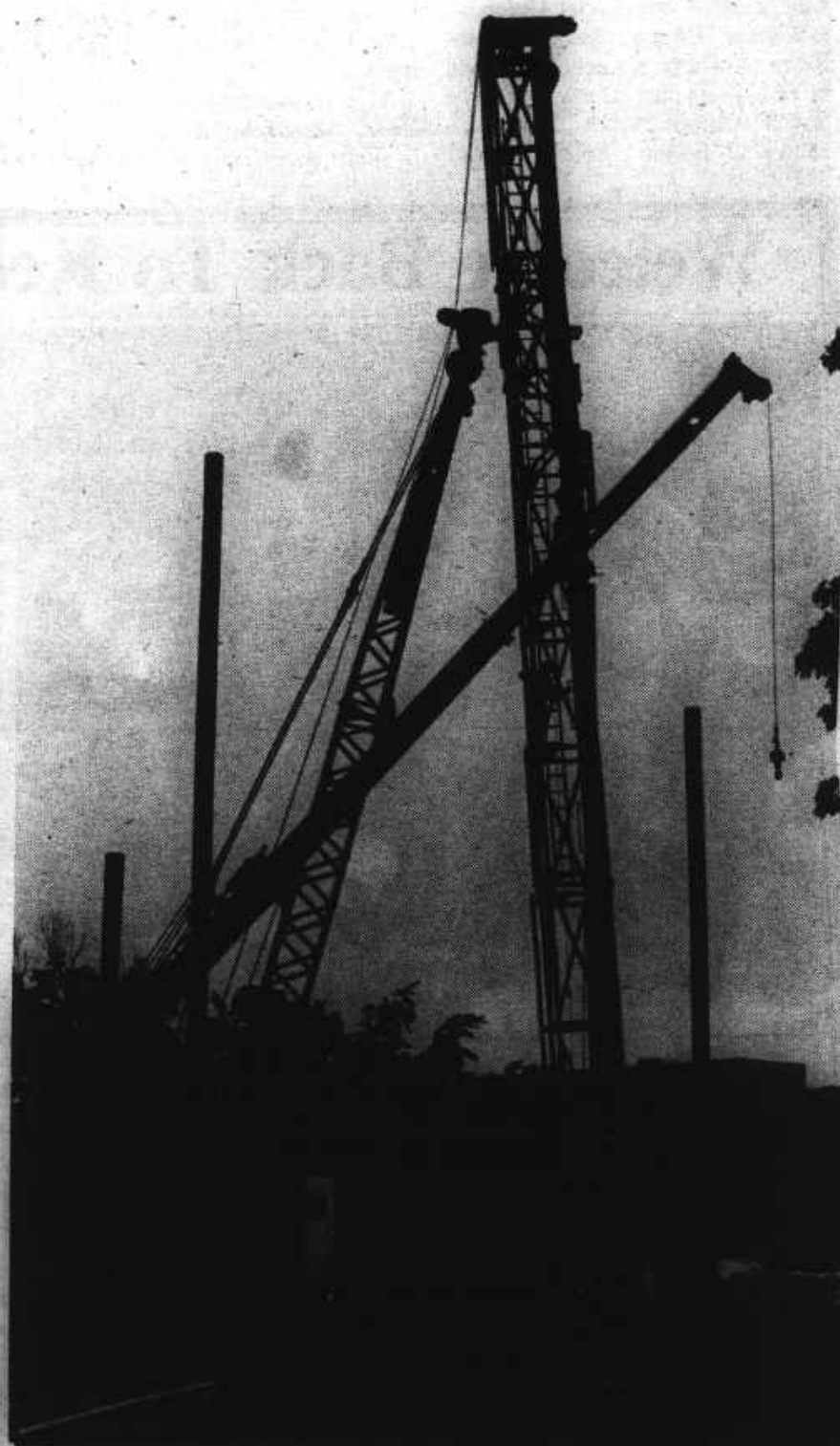
Construction continues as workers from H. Loney Construction Co. drive piles at the site of the new residence hall.
