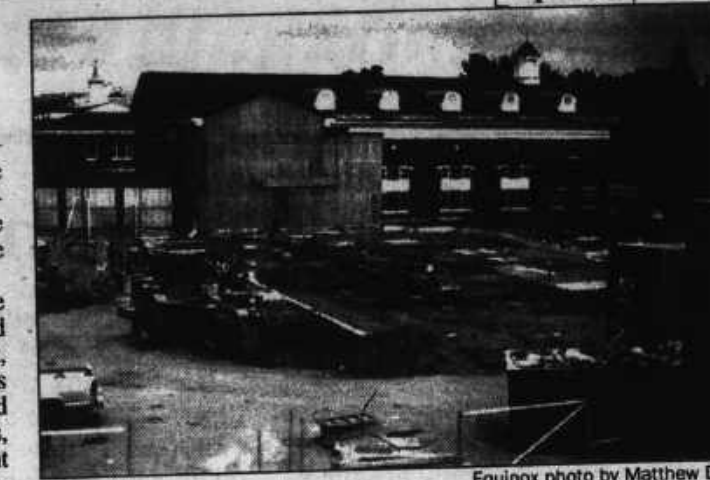
Equinox photo by Matthew Daly Construction crews have been working diligently to finish the foundation of the Rhodes Hall addition.
