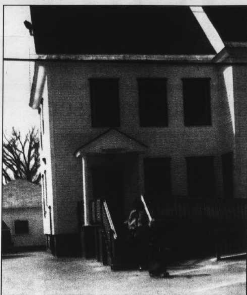
Students will be finding their professors' offices in the library during the renovations to the math center.
